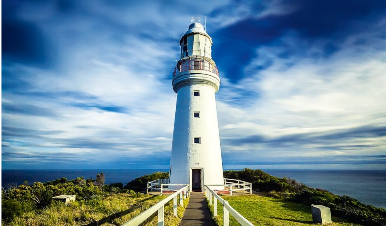
Cape Otway Lightstation, Great Ocean Road, Victoria.
